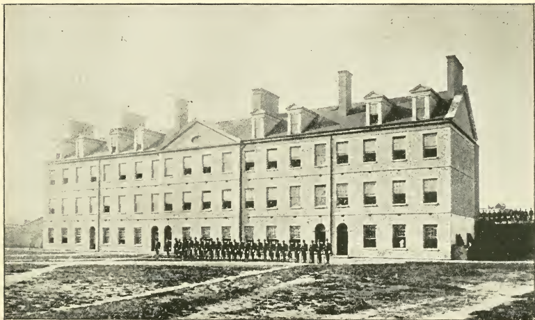
BARRACKS, FORT WAYNE.
