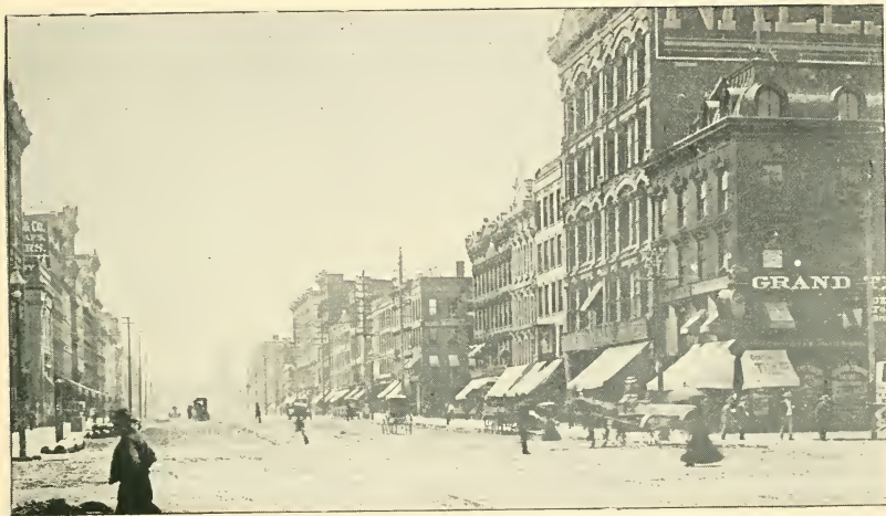
STREET VIEW, LOOKING WEST ON JEFFERSON AVENUE, FROM WOODWARD AVENUE.
