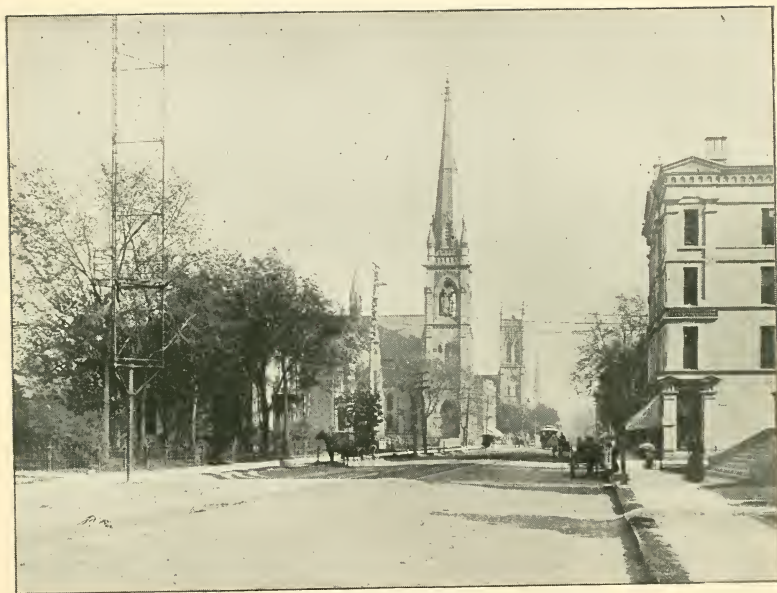
STREET VIEW, LOOKING SOUTH ON WOODWARD AVENUE, FROM ADELAIDE STREET.
