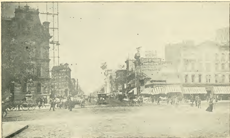
STREET VIEW, LOOKING WEST ON MICHIGAN AVENUE, FROM WOODWARD AVENUE.
